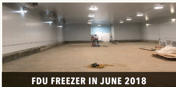
FDU FREEZER BEFORE CONSTRUCTION
