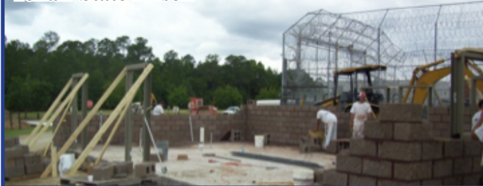
Front Bunker Construction Telfair State Prison
